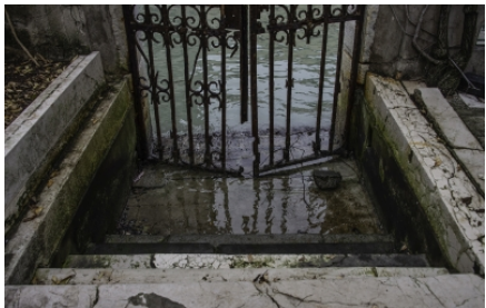
Abandoned Canal Gate Venice Acceptance Frances Cunningham
